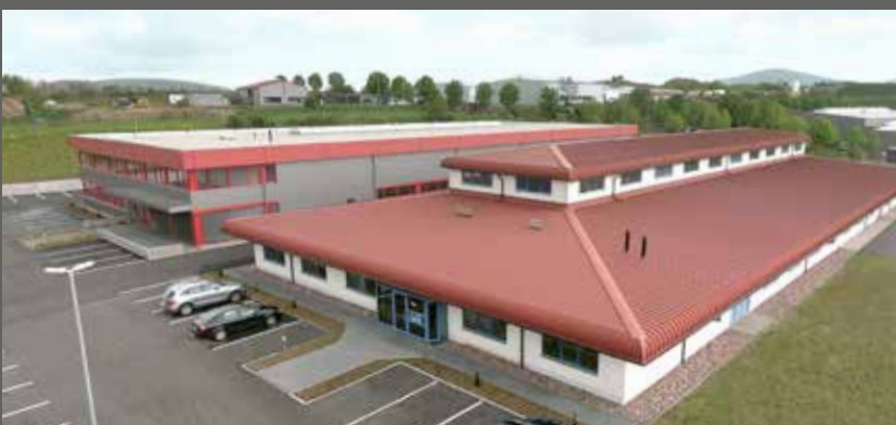
Plant in Eiterfeld
